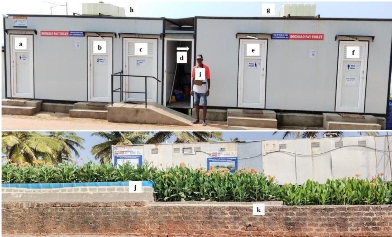
Fig. 1 Public toilet with decentralized integrated treatment system at Bogmalo beach, Goa-India (a) Changing room, (b) Female toilet, (c) Handicap toilet, (d) Electro-chlorinator room (EC), (e) Male toilet, (f) Male urinal, (g & h) Fresh water tank, (i) Toilet keeper, (j) 1 st stage unsaturated- vertical flow constructed wetland (U-VFCW) (k) 2 nd stage saturated- vertical flow constructed wetland (S-VFCW)
