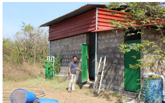
Biogas bag and Compressor Room
