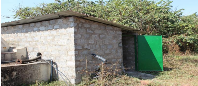
Food waste Macerator room
